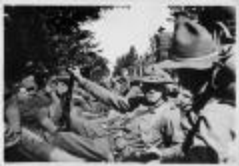
Men in Trench (NYSA_A0412-78_B09_F10_Men_trench)
