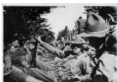
Men in Trench (NYSA_A0412-78_B09_F10_Men_trench)
