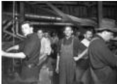
Hat factory: finishing room with ducts and fans (NYSA_A3029-78_B5_F3)
