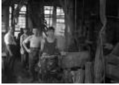
Hat factory: scalding room, felt hat making (NYSA_A3029-78_B5_F2)
