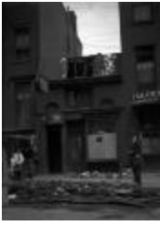
Exterior of Oxyozon Disinfecting Co. after fire (NYS A3029-78_B3_F4)
