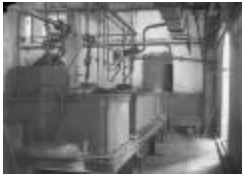
Interior of factory room with large vats (NYSA_A3029-78_B2_F10)
