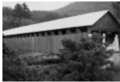
Blenheim Bridge in North Blenheim, New York (NYSA_A0245- 77_Schoharie_B20_34_A)
