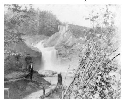
Canal Break at Forestport. This is judged to be but a few hours after the banks were cut through on top, the water of canal still rushing through.
