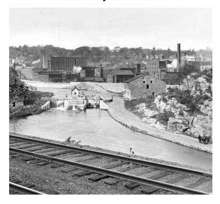
New York. Old Erie Canal. Double locks side by side; one filled with water, the other containing boat at lower water level. Little Falls. (1911)
