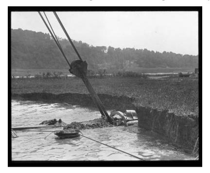
View of a cutter head of a dredge working against a bank on the Champlain Branch of the New York State Barge Canal, somewhere in Washington County.
