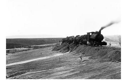
New York. Barge Canal. Unloading dump cars to make fill across Irondequoit Valley. East of Rochester. (1910)
