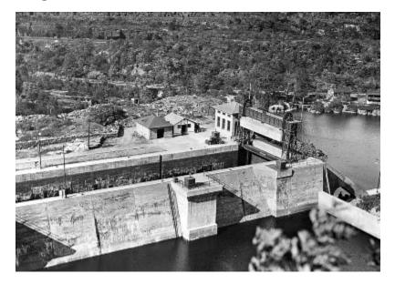
New York. Barge Canal side view of Lock 17 from Hillside: concrete masonry, side pool and powerhouse. Little Falls. (1921)
