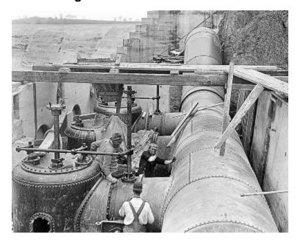
New York. Barge Canal. Double guard gate. Pendleton. Workers installing turbines. (1913)
