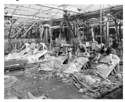
Several men bending over animal hides over a board using a hand scraping tool to remove matter from the skins. Scrapings cover the floor. Behond the men, large belts suspended from the ceiling power tanning equipment. Endicott Johnson Plant, Endicott, NY, (1917).
