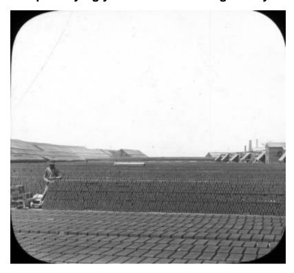
A man stacks bricks in the drying yard of a brickmaking facility in Haverstraw, New York. Rows of bricks extend into the distance, filling a large yard lined with buildings on either side. Smokestacks protrude from buildings on the right. Lantern slide is cracked.
