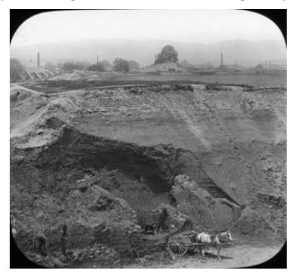
A lonely horse pulling a loaded cart stands beside a high clay bank at the excavation site of a brickmaking facility in Haverstraw, New York. In the background are buildings with smokestacks. Hills rise in the far background.
