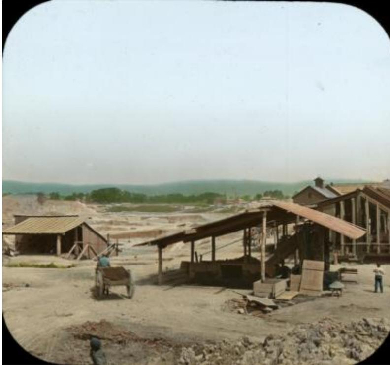
Exterior view of moulding machine under an open shed at a brickmaking facility near Haverstraw, New York. A worker drives by with a cart loaded with clay. More sheds and buildings are visible in the background.
