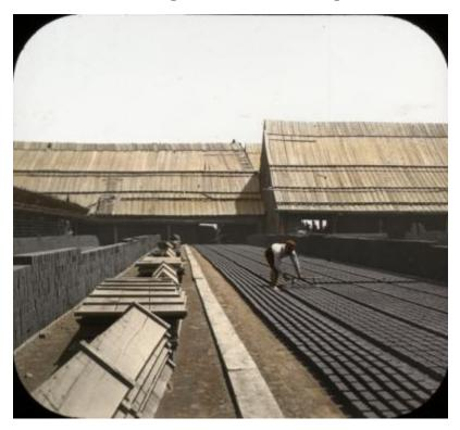
A workman turns rows of soft bricks on their edges in the drying yard of a brickmaking facility near Haverstraw, New York. On the left are stacks of drying pallets and rows of stacked bricks. Men work in open sheds in the background.
