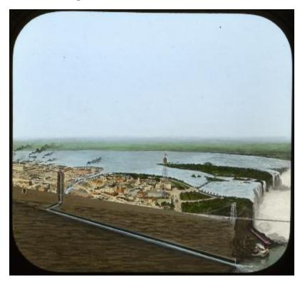
Panoramic drawing of Niagara Falls showing a plan for an electric power plant above the falls. The power plant is drawn as part of the town of Niagara Falls on the shore of the Niagara River above the falls. In the foreground, the drawing shows a cross-section of the ground underneath the power plant, revealing a tunnel of water passing underground from the power plant to the river below the falls.
