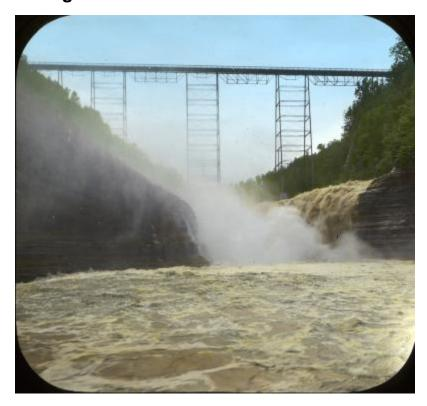
View from below of the Upper Falls and railroad bridge on the Genesee River in current-day Letchworth State Park near Portageville, New York. The iron bridge was a replacement for the Portage Wooden High Bridge that claimed to be the highest wooden bridge in the world at the time. The iron bridge was completed in the 1870's after the wooden bridge was destroyed by fire.
