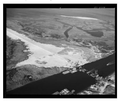
View of a line of pilings being set into a narrow channel between two islands (Captree Island and Oak Beach) as part of the construction of the Captree State Parkway Bridge (later renamed the Robert Moses Causeway) linking Fire Island to West Bay Shore in Islip, Suffolk County. The bridge opened in 1954.
