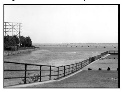
View of a hydraulic canal at its junction with the Niagara River. The canal diverts water from the river for industrial purposes. The opposite shore of the Niagara River is visible in the far background.
