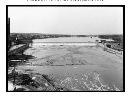
View up the Hudson River at Mechanicville, Saratoga County showing a dam, Champlain Canal Lock No. 3 (right), and what is either a headrace (a waterway that feeds water to a mill, water wheel, or turbine) or a fore bay (a reservoir between a mill race and a water wheel) (left).
