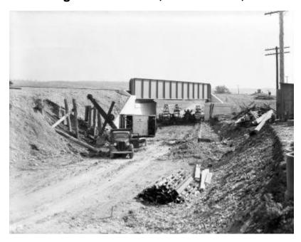
Road work under a new bridge (possibly railroad) in a rural area of Cattaraugus County. A cable shovel excavates an embankment; several trucks, crewmen, equipment, and the roof of a nearby building are also in view. The project is associated with Public Service Commission number 5335. The image is a construction progress photograph taken by the Dept. of Public Works (related photograph file number 1435).
