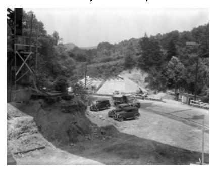
A highway underpass being constructed in a hilly, wooded area of Orange County. A crane, dump truck loaded with gravel, three cars, and workmen are also in view. Project is described with "W.P.G.H. - RC#3686". The image is a construction progress photograph taken by the Dept. of Public Works (related photograph file number 1277).
