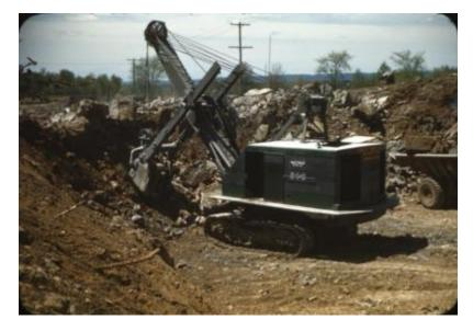
Cable shovel digging earth and rock at a highway project site. Image is a construction progress photograph of the Dept. of Public Works project FARC 47-64; Broadalbin - East Galway, state highway 8045 (related photograph file no. 4644).
