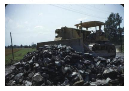
Workman operating a bulldozer moving rock fill. Image is a construction progress photograph of the Dept. of Public Works project RC47-138, state highway 1345, Mechanicville – Clifton Park, state highway 4712, Crescent–Mechanicville. Sta. R123, rock fill (related photograph file no. 4718).
