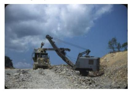
Cable shovel loading earth and rock into a dump truck. Image is a construction progress photograph of the Dept. of Public Works project RC47-138, state highway excavation in Mechanicville and Clifton Park (related photograph file no. 4718).
