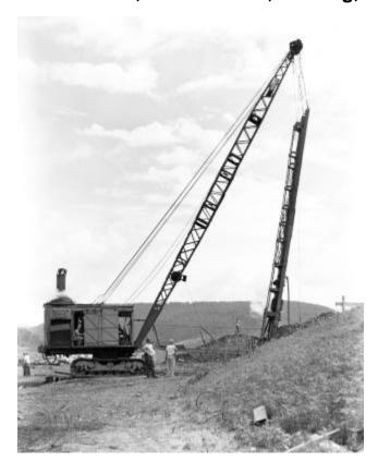
Workman operating a Bucyrus Erie steam powered crawler crane to drive piles at east abutment of the Cutler Creek Bridge. The work is Public Service Commission project number 9418 (Sta. 50' west of east abutment of Cutler Creek bridge and 100' right of center line, L. N.E). The image is a construction progress photograph taken for the Dept. of Public Works, Bureau of Bridge and Grade Crossings (related photograph file 5233).
