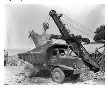
Cable shovel loading earth and rock into a dump truck, owned by John Arborio, Inc., Poughkeepsie, N.Y., during a state highway construction project, Mechanicville to Clifton Park (SH 4712). The image is a construction progress photograph taken by the Dept. of Public Works (related photograph file number 4718).
