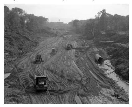
View overlooking workmen operating tractors, dump trucks, and bulldozers, excavating a wooded area for the Thruway. A three-story building and water tower can be seen in the background. The image is a construction progress photograph taken by the Dept. of Public Works, Bureau of Highways (related photograph file number 5651).
