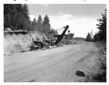
A cable shovel, owned by Mayersohn Construction, Albany, NY, loading rock into a dump truck at a road construction site in the Adirondacks, possibly Route 28N. The image is a construction progress photograph taken for the Dept. of Public Works, Bureau of Highways (related photograph file 6919).
