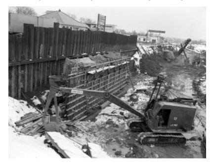
Two Link-Belt cable shovels at an excavation site near the Crossroads Restaurant and Latham Rug Company (signs visible) in Latham, NY. Crewmen can be seen working on and around cable shovels. The image is a construction progress photograph taken for the Dept. of Public Works, Bureau of Highways (related photograph file 7120).
