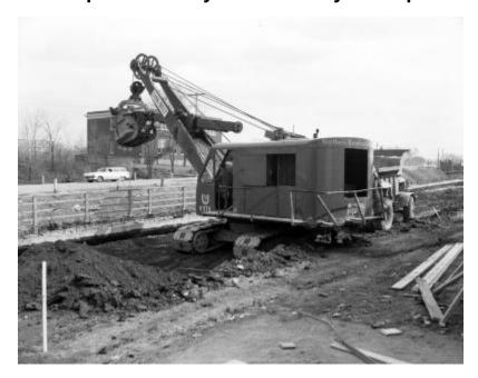
A Link-Belt cable shovel (Northern Construction visible on cab) and a dump truck excavating alongside a highway, probably in Latham, NY. A two-story brick building sits across the highway in the background; cars are also in view. The image is a construction progress photograph taken for the Dept. of Public Works, Bureau of Highways (related photograph file 7144).
