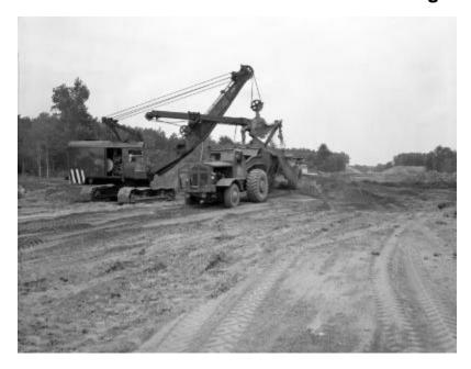
Cable shovel loading dirt into dump trucks at an excavation site in a wooded area of Saratoga County. The image is a construction progress photograph taken for the Dept. of Public Works, Bureau of Bridges and Railroad Grade Crossings (related photograph file 7220).
