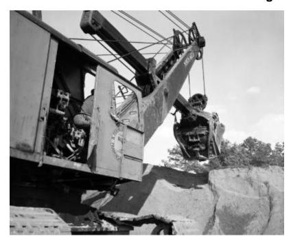
Detail of a workman operating a cable shovel owned by B. Perini and Sons, Framingham, Mass. The image is a construction progress photograph taken by the Dept. of Public Works, Bureau of Bridges and Grade Crossings (related photograph file number 7274).
