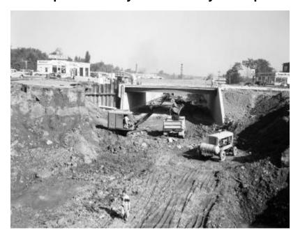
View of a construction site at an overpass in Latham, NY, including a Mobil Station, Sherwin-Williams Paint, and Thunderbird Motor Hotel. A cable shovel loading a dump truck, workmen, and other heavy equipment are in view above and below the overpass. The image is a construction progress photograph taken for the Dept. of Public Works, Bureau of Highways (related photograph file 7290).
