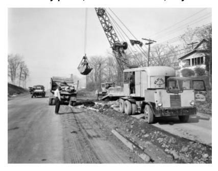
Workmen operating a crane (owned by Kilby Bros., Inc., Albany, NY), a bulldozer, and dump truck scrape up and haul slabs of roadway from a site in a residential area of Watervliet. Houses and a utility truck are also in view. The image is a construction progress photograph taken for the Dept. of Public Works, Bureau of Highways (related photograph file 7325).
