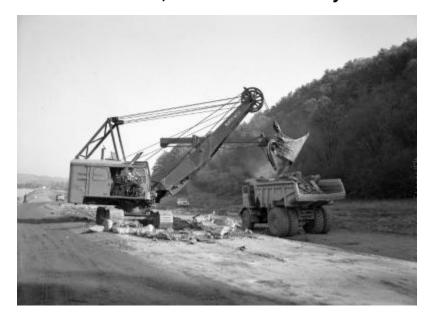
Workman operating a Northwest cable shovel, loading pieces of old roadway into a dump truck on a long stretch of highway, possibly NY Route 22. Trucks, crewman, wooded areas, farmland and low hills are in the background. The image is a construction progress photograph taken by the Dept. of Public Works, Bureau of Highways (related photograph file number 8737).
