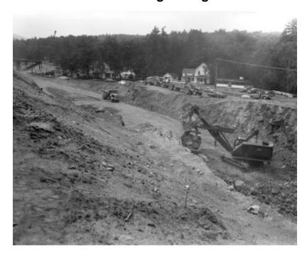
View overlooking an area in Lake George Village excavated for a new road, probably Route 9. Workmen, a crawler cable shovel, three dump trucks, a utility truck, cars, houses, Family Diner, and Dwarf's Motor Court are in view. A bridge overpass and the Adirondack forest are in the background. The image is a construction progress photograph taken by the Dept. of Public Works (related photograph file number 8948).
