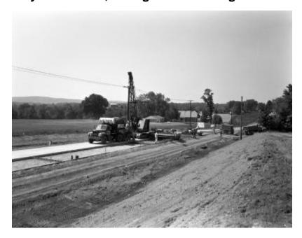
Workmen paving a road, probably Valley Falls Road in Schaghticoke, Rensselaer County. The road crew, a Latham Concrete truck, a crane, and dump trucks are in the foreground and several farms can be seen in the background. The image is a construction progress photograph taken by the Dept. of Public Works (related photograph file number 8984).
