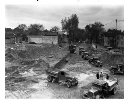
Railroad construction, possibly on South Main Street in Elmira. A crawler crane is digging up the street and several workmen and trucks are on site. A sign for Keefe Grocery Co. is on one of the buildings along the residential tree-lined street in the background. The project is associated with Public Service Commission number 3200. The image is a construction progress photograph taken by the Dept. of Public Works (related photograph file number 1031).
