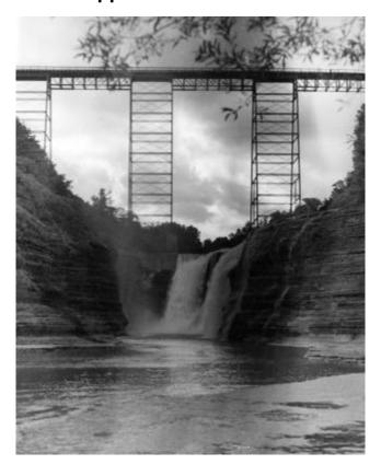
Photograph of the Erie Railroad Bridge over the Upper Falls of the Genesee River in Letchworth Park. This wooden trestle bridge was built by the Erie Railroad Company over the Genesee River. The bridge was built between 1851 and 1852. The wooden bridge was destroyed in a fire in 1875, but was replaced with an iron and steel bridge in the same year.
