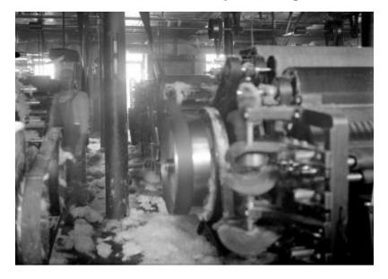
A workman stands beside machinery for carding cotton at the Washington St. plant of Union Mills, a men's underwear manufacturer in Hudson, New York. Cotton floss covers the floor, clings to machinery, and fills the air. An investigator noted the need for exhaust fans that would remove the floss and reduce the risk of fire.
