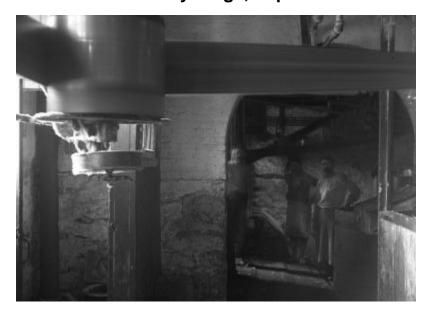
Interior of cellar of Union Mills, a men's underwear factory on Fulton St. in Hudson, New York. Three men stand beyond an arched doorway next to large rolls of white cloth being fed into a machine. Overhead, large transmission belts less than six feet from the ground lack protective guards.
