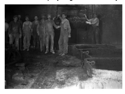
Workmen at The Waterbury Wire Cable Manufacturing Co. in Brooklyn, New York, stand next to a coil of wire rope suspended from the ceiling. Machinery lacks protective guards. The men's clothing appears to be covered with a chalky substance, which is also visible on the floor.
