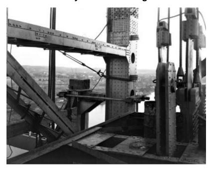
Closing of span during the construction of the Troy-Menands Bridge. Work was done by the engineering firm F.J. Hart and J. A. McMahon.
