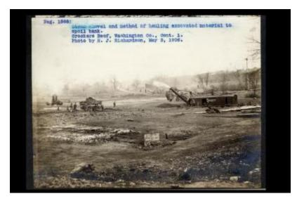
Contract 1. Steam shovel and method of hauling excavated material to spoil bank. Crocker's Reef, Washington County. Photographer H. J. Richardson, May 3, 1906.
