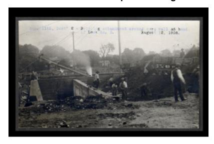
Contract 2. A view of workers building an embankment around the core wall at the head of Lock 3.
