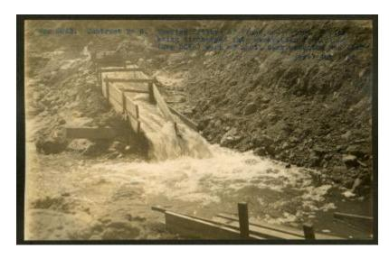
Contract 6. An image showing the failure of a flume and the volume of water being discharged into excavation from the flood. The image was taken from west of the Spoil Bank, opposite Station 2622.
