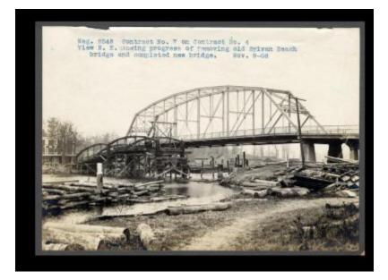
Contract 7 (on Contract 4). A view from the northeast showing the progress on removing the old Sylvan Beach Bridge and the completed new bridge.
