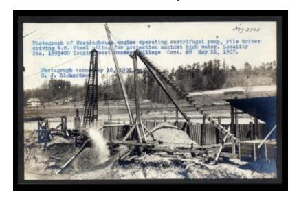
Contract 8. A photograph of a Westinghouse engine operating centrifugal pump, a pile driver driving W.S. Steel piling for protection against high water that was taken by H.J. Richardson. Locality Station 1993+00 looking west Cranes Village [Cranesville?].
