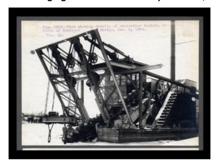
Contract 12. A view showing details of excavation buckets on the front of a conveyor and dredge.
